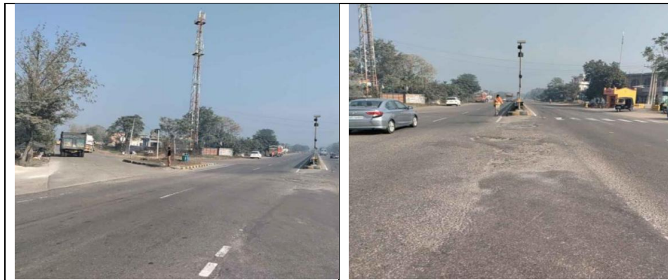
Fig.5: Blackspot Location T-Point Malikpur.
